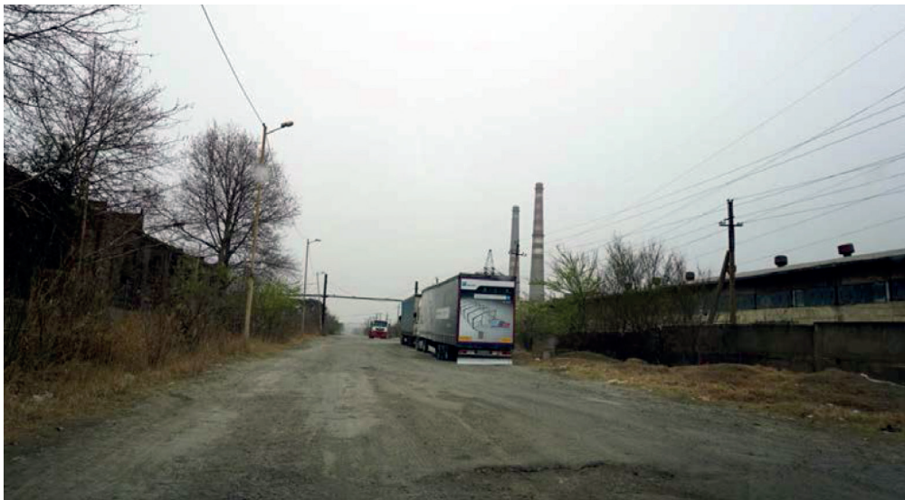
Enterprise “Geosteel” - unarranged road surface near the administrative building.
